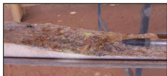
Open joint with some uranium oxides from Tchirezrine II unit at Imouraren site (Orano Internal Report).
