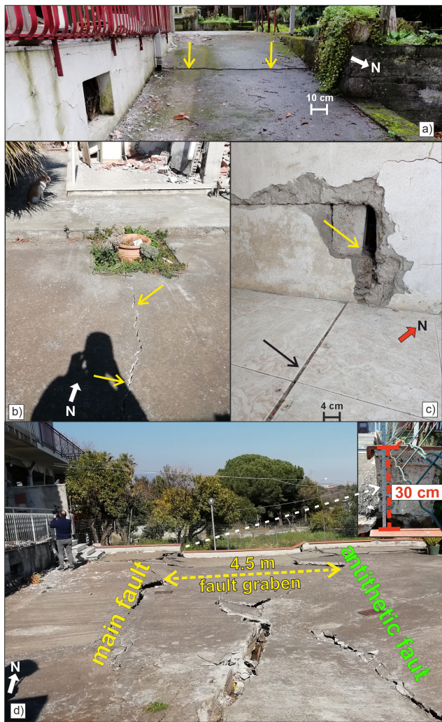
Figure 5. 26 December 2018 coseismic ruptures at Fiandaca trench site (see photos location in Fig. 4): (a) ground rupture along a private road with few cm of offset; (b) ground rupture which follows a damaged building wall, offset ~1 cm; (c) 1.5 cm horizontal offset between two floor tiles continuing into the wall; (d) fault graben on a private asphalt parking which extends over the wall and farmland. Photos taken on: 26 December 2018 (a); 22 January 2019 (b and c); 18 February 2019 (d).
