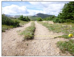
Secondary treads are more common in areas with lower grade - Ute West Trail.
