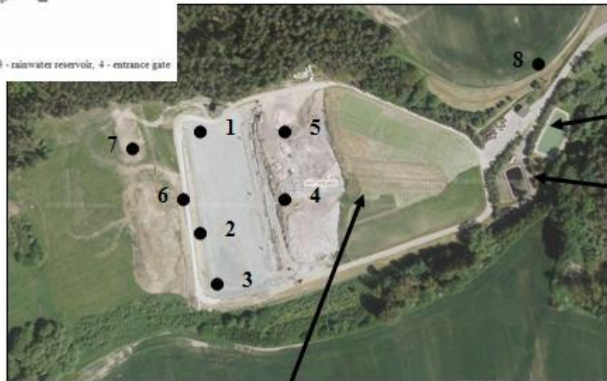
Section of the landfill
