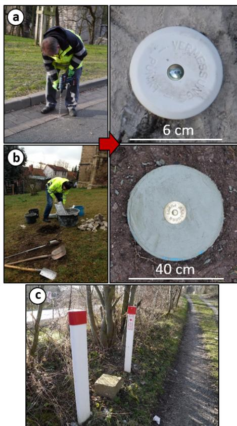
**Figure 4.** Installation of the time-lapse measurement network - (a) Drilling of levelling/gravity points that were stabilized by 30 cm long steel piles and marked by synthetic survey markers. (b) Pouring of an 80 cm deep concrete base with even surface and brass survey markers. (c) Example of benchmark RP1 provided by the Thuringian State Office for Surveying and Geoinformation (TLVermGEO, pers. communication, 2013).
