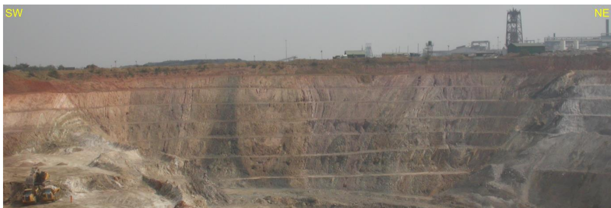
5 Figure 9: Cross-section view towards the northwest side of the Nkana South open pit, taken August 14th 2012. The COM is the black layer, showing isoclinal folding and pinched out fold hinges. Compare with Fig. 8B for geology in cross-section.
