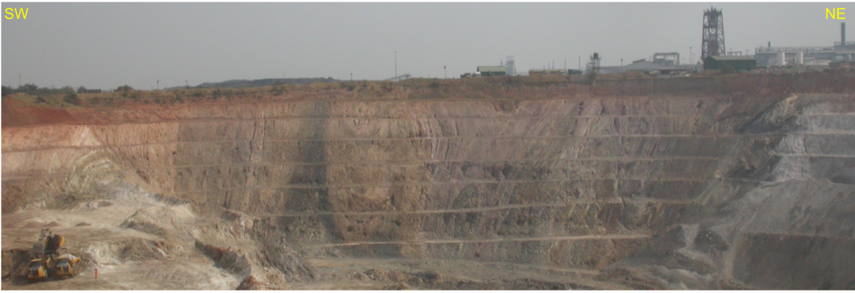
Figure 9: Cross-section view towards the northwest side of the Nkana South open pit, taken August 14th 2012. The COM is the black layer, showing isoclinal folding and pinched out fold hinges. Compare with Fig. 8B for geology in cross-section.
