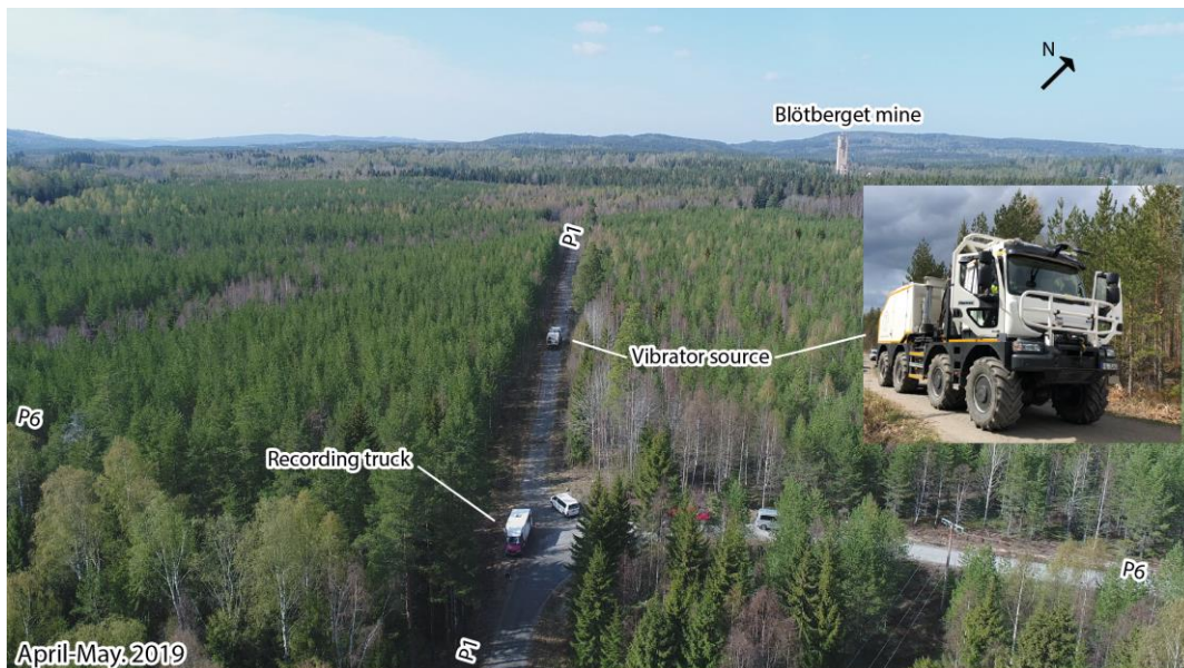
Figure 3. Field photos from the 3D seismic survey (April-May 2019) in the Blötberget mine. The survey was conducted using the 32t vibrator of TU Bergakademie Freiberg, 1266 receivers of which 414 were cabled (part of P1 and entire P3). The cabled profiles were used for live data quality control and sweep parameter tests. Earlier reported 2D profiles (years 2015 and 2016) were also along P1. Photos by Alireza Malehmir.
