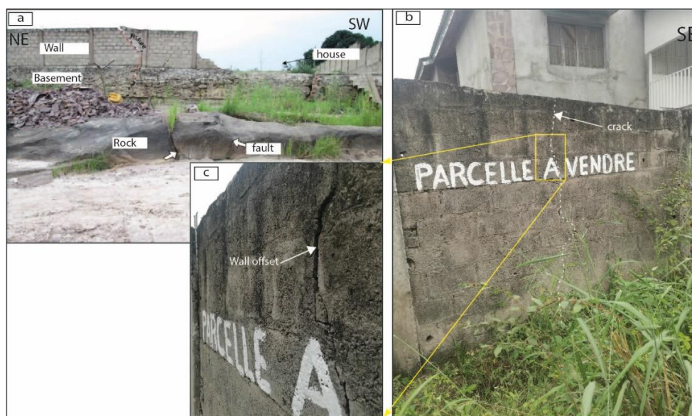
170 Figure 6 : Home linear breaks. (a) Linear breaking of a fence in parallel direction with faults in the sandstones of the Inkisi sandstones. Fractures even affect the foundation of the fence. (b) Home placed for sale due to the appearance of linear breaks (c) A lateral movement along the wall of the fence.
