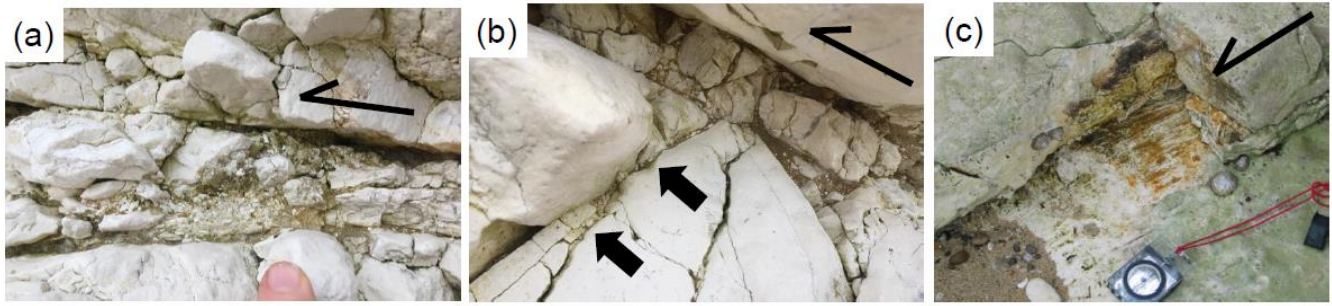
Figure 64. Structures associated with contractional structures in Selwicks Bay; all from locality 3 . (a) Crush breccia along top-to-the-S thrust fault reoriented by later, normal fault-related tilting. (b) Crush breccia and brown gouge derived from chalk and shale, respectively, associated with top-to-the-S thrust fault with narrow gouge injections into footwall, one of which is arrowed.
